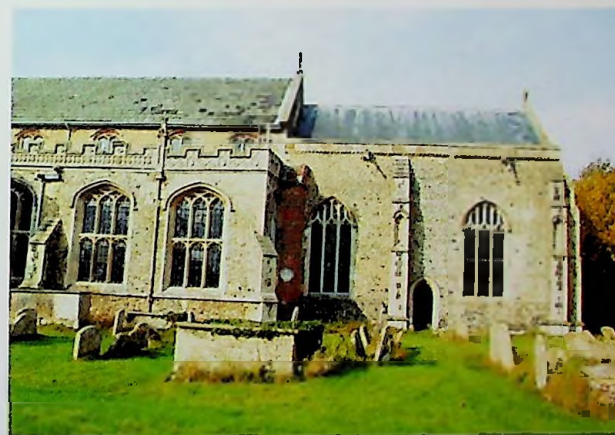
the churchyard, chancel and the south aisle, showing the parapet, with its rich carving, and the external casing of the rood stair.
