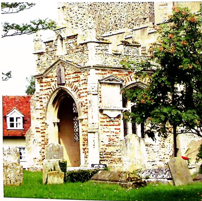
The south porch. ©
