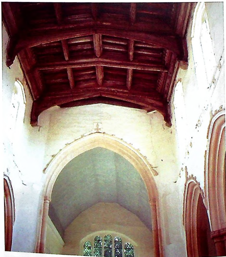
East end of the rebuilt, late-15th-century nave with low-cambered roof and clerestory. ©
