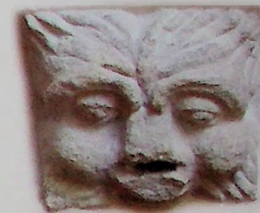
A detail around the vestry door.
