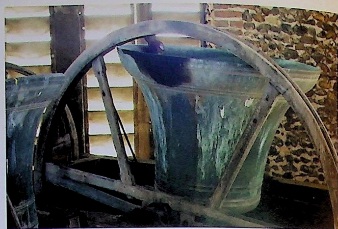
6 th (tenor) Bell in the up position, ready for ringing
