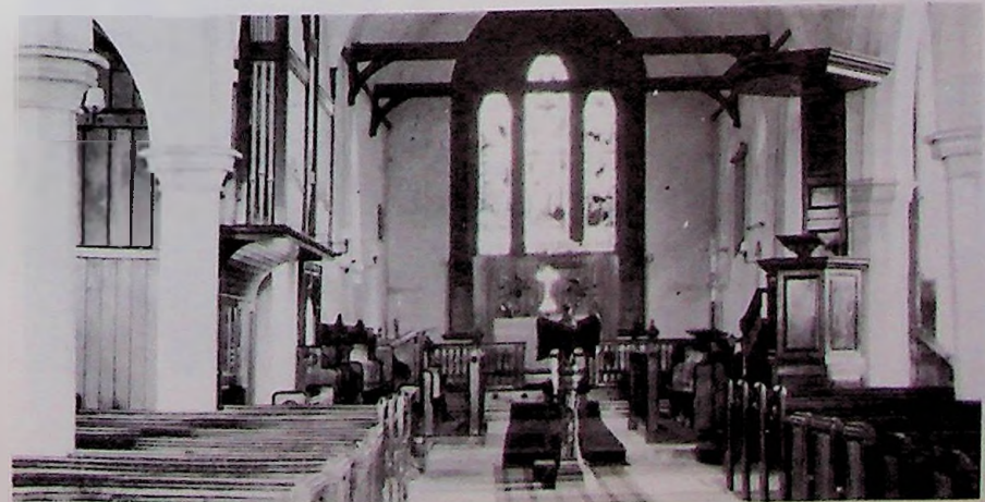
(below) Interior of Exning Church — taken before the organ was moved to the west end
